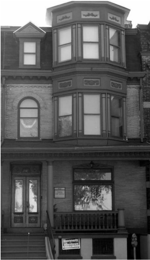
FIGURE 3. Building with a high degree of historic integrity.
